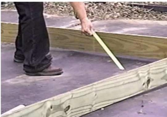
**Shift side "B" left or right until you get five feet between the two marks on the diagonal measurement. It's then square, Provided that you have cut all four of the side boards to their required length, if one board is wrong then the frame will not square up...**
