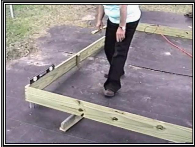
**As you can see we have already installed the ground cloth in a large area inside and out side of greenhouse. The ground is sloping towards this corner. After installing the 1 5/8 inch ground stakes I leveled the wood frame then blocked the frame up where needed to keep it level. Next step is to install the hoops.**
