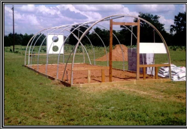
**Another customer supplied photo. A great example of a very clean professional job preformed by the homeowner. Note the holes for twin exhaust fans in rear. He used tubing framing for end walls but bolted wood to front end wall for easier door installing.**
