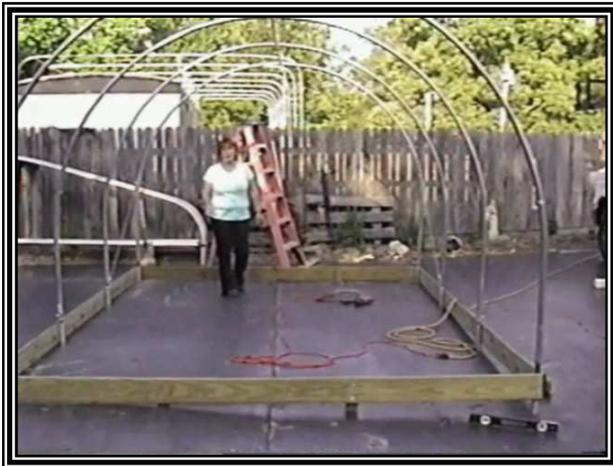
**The gap at front right corner will be filled in with treated wood later, leaving a screened outlet hole for water to escape the greenhouse.**
