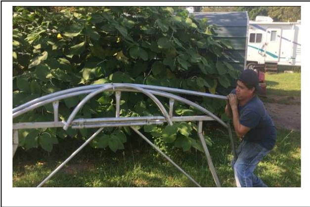
Add the lever bar to the swaged (small) end
