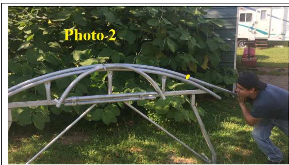
Position the two tubes you bent, one against the right side 2x4 and the other against the left side 2x4 as shown in photos 4 & 5
