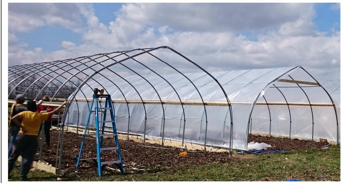
***You are building the Template Hoop, after it is completed all tubing can be precut and remaining hoops assembled on top of this template hoop, one at a time. Don't build and stack multiple hoops on top of the template***
