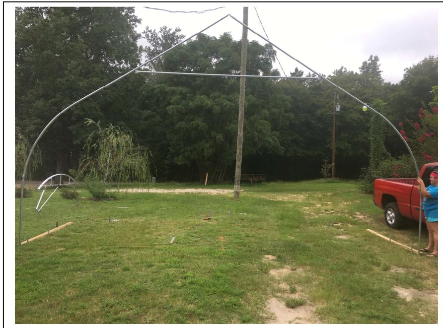
Here is a side view of a 24x120 frame setup bolted to the 1 5/8" anchor post stakes and top purlin installed. The two side purlin have not been installed yet. Their relative locations can vary a foot or two from the location demonstrated in photo below.
