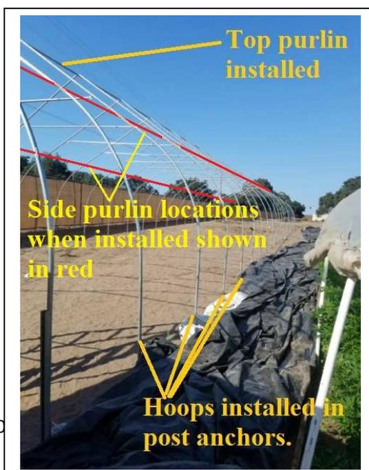
Anchor post are made from 1 5/8" od fence post in 15, 16 gage wall thickness.
