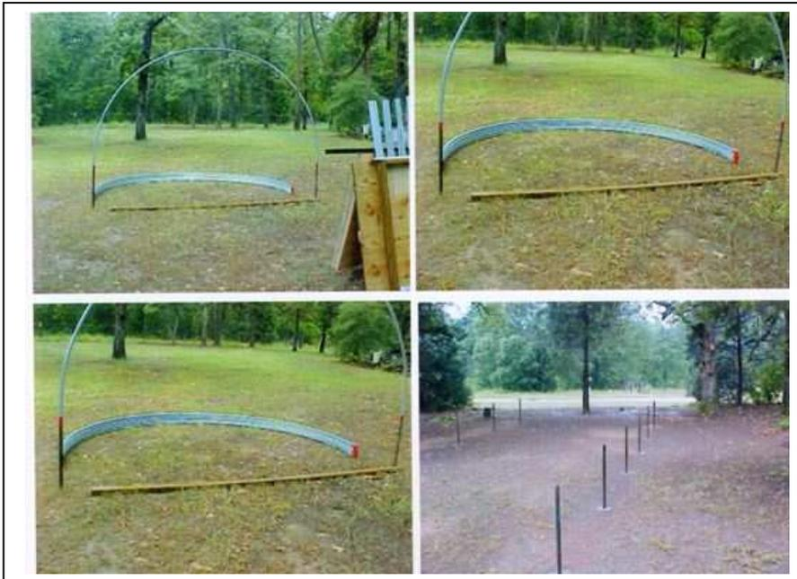
Side purlins are attached at each end of the greenhouse using the purlin end adapters. Or you can make you own by flattening the end of the purlin, bending it upwards to about 30 degrees as shown in this photo.
