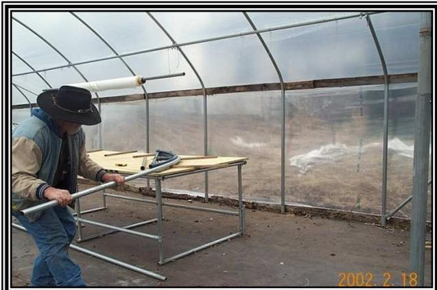
Here I'm completing the final bend on one section for a 16 foot hoop. Note the already bent tubing being supported at the opposite end with the 1"x2" wood strips
