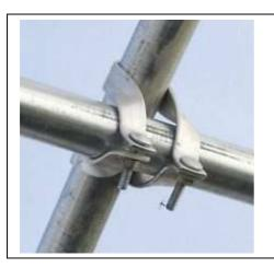
However we recommend using factory purlin clamps on greenhouse especially larger 16 ft or wider houses
