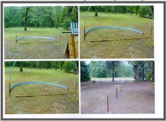
An alternate method for smaller in ground anchored greenhouses is simply build a sand box with 2x4s, level it, square it, then drive the stakes inside the sand box, using the box as a guide for stake spacing and alignment. Install hoops in stakes, fasten with tech screws from inside the greenhouse opposite the 2x4. After hoops are installed drill through the 2x4, stake & hoop and bolt them all together using 1/4"x4" carriage bolts or skip the drilling and use longer tech screws
