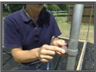
Here we are using those handy 1 3/8" fence band clamps. Any chain link fence supply can order these clamps if you can't find them. Also some success has been noted using heavy metal plumbers tape with holes punches in it. Or solid tubing braces can be used, cut the tubing to desire length flatten the ends and tech screw it to the inside of hoops at the four corners. In place of the cables
