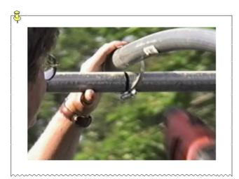
A simple stainless steel hose clamp is used to connect all hoops to the purlin except for each end hoop, which is bolted.
