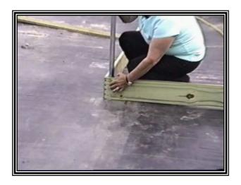
Install the self drilling (Tech) screws from outside wood into the 1 5/8" stake and hoop
