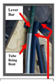
Every bending stroke should end about 5 inches from the end of the bender
