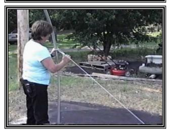
Here we are attaching cable to the end hoop at one end. Tighten the band clamp securely on the lower cable end at left and just sung up the band clamp at end hoop, leave some slack it cable for now. Install cables on opposite end same way
