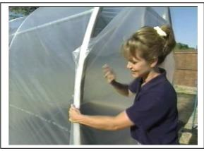
There are many different Poly Latching systems on the market from Wiggle Wire poly lock to Aluminum track lock. Most all of these must be installed over the top of wood frame for strength. Snap clamps are only recommended for smaller 10x10 or 12x12 portable garden units and are not recommended for larger in ground units. For use of our plastic snap clamps on small units please refer the specific unit you are building.
