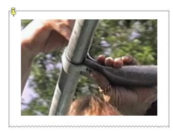
Attach the purlin at each end by flattening out the ends then bending the flat portion of tubing up about 30 degrees, drilling a 5/16 hole and using a band clamp made for 1 3/8" fence tubing. If you can not locate these fence clamps just make the purlin 1 3/8" longer on each end, flatten as shown, Holding the flat portion under the hoop and drill 5/16 hole thru the hoop and flatten end of purlin, then bolt with 2" X 5/16 bolt.
