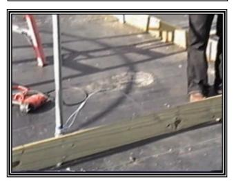
Here the cable brace has been clamped securely to the bottom of the first hoop back from each corner.
