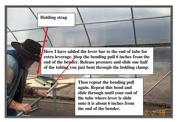
Always start the bending with the painted ends of both sections inserted through the holding strap twenty four (24 inches). In the case of bending never place the un-pained ends into holding strap first when bending these 10 ft hoop sections.
