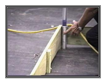
Pushing the hoop down into the 1 5/8" O.D ground stake. Here you can see the top of painted end. Top of paint is 6"
