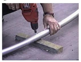
You can also stand the hoop sections up against the side of a building then connect the joints with tech (self drilling) screws same as shown in the photo above (right) if you were using the flat ground method for assembly. Using the side of a building is a very good method if a suitable one is nearby
