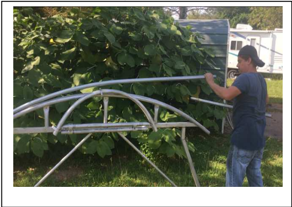
Add the lever bar to the swaged (small) end
